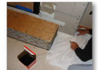
Building a new hearth out of plywood, followed by wire mesh, anchoring to floor, scratchcoat, then stone.
